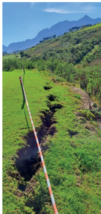
The downpours cut dongas into the earth surrounding a bunker face.
